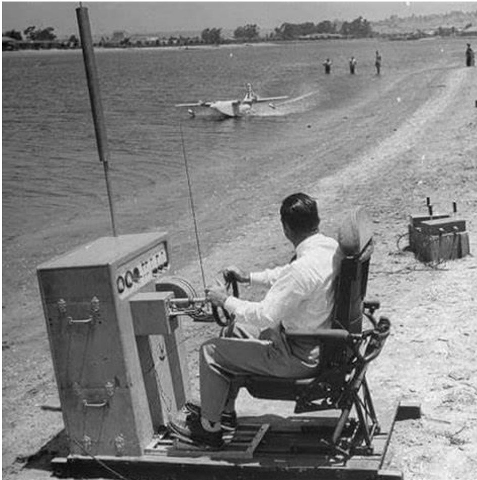
Howard Hughes test flying (taxing) a radio control scale model of the HK-1 (Spruce Goose) from his large remote controlled consol, circa 1940.
