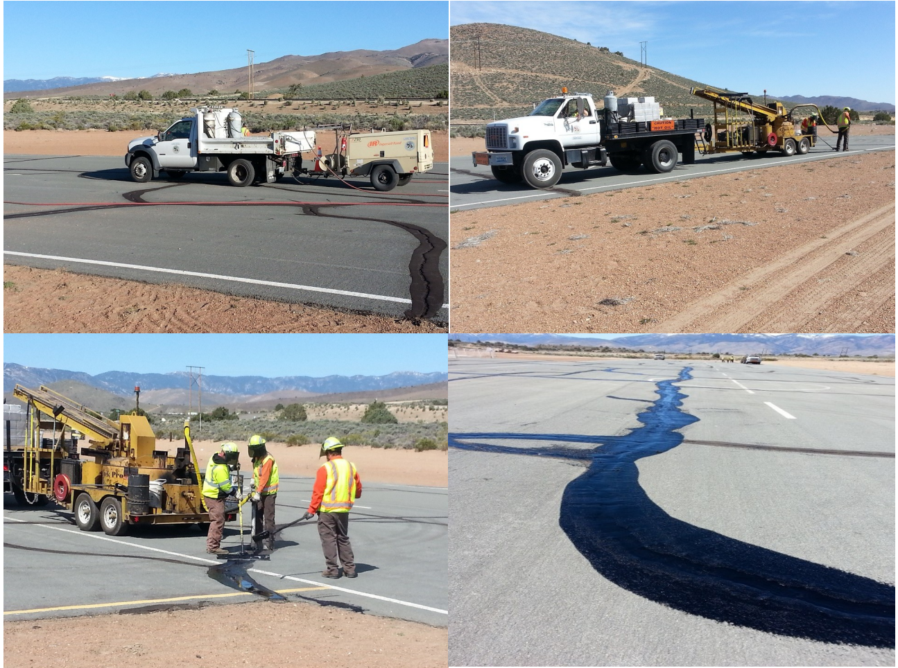
Carson City crews finished repairing the surface of the runway.
